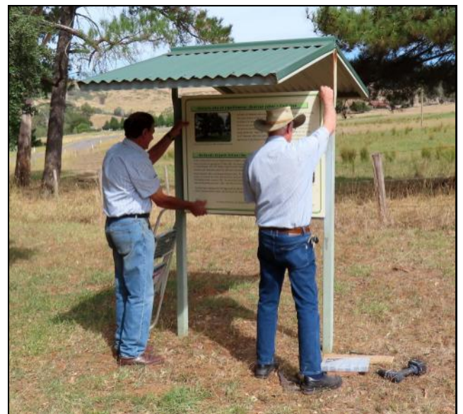
Greg & Joe erecting the sign
